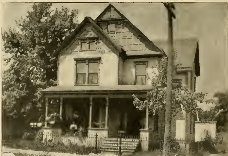
RESIDENCE OF PROF. J. D. COLLINS. South 5th Street.
